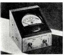
ulated carrier, as well as giving an indication of carrier shift. It enables the user to avoid over-modulation.
